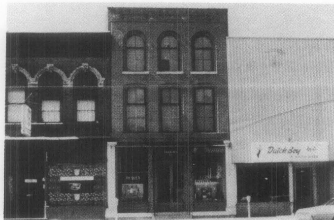
Figure 12. This photograph of three late 19th century commercial buildings clearly shows the impact of preserving and rehabilitating storefronts. The one on the right has been totally obscured by a "modern" front added in the 1950's. Although inappropriate alterations have taken place on the left storefront, it is still possible to determine the original configuration of the doors and display windows. The storefront in the middle has remained intact. Although in need of some minor maintenance work, the appeal of the original design and materials is immediately apparent.
