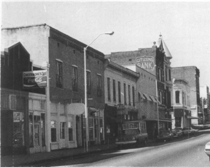
Figure 1. Inappropriate storefront alterations over the years—metal cladding, oversized signs and canopies—have detracted from the character of this historic district in Van Buren, Arkansas. A carefully considered rehabilitation plan for Main Street, including the removal of poorly designed signs, false fronts and the selection of an appropriate exterior paint color palette, serves to enhance the visual environment and preserves the district's sense of time and place. Photo above: Bob Dunn; Drawing, David Fitts
