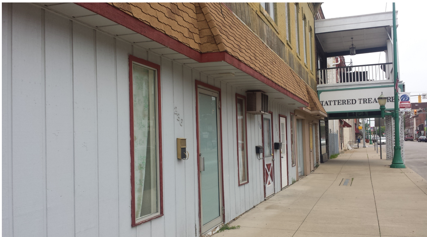
Wood siding, asphalt shingled awning, and inappropriate doors and windows should be removed.
